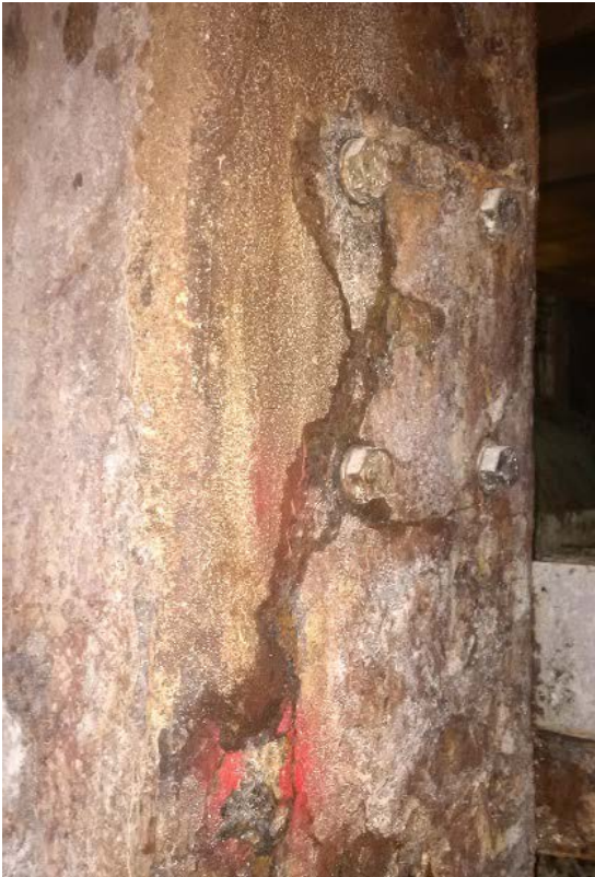
Wire section framing corroded especially on drive side
