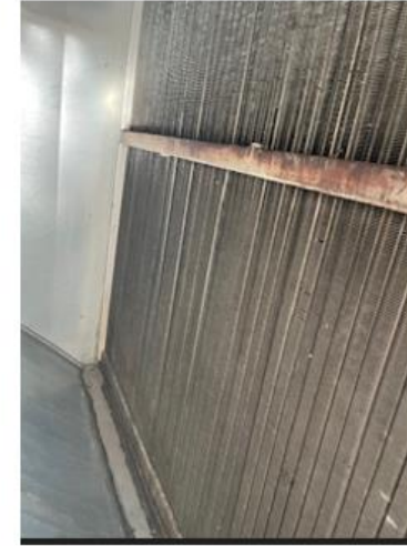
CASE2. Improved air flow with cleaning of the plugged filter for the supply air V2906
