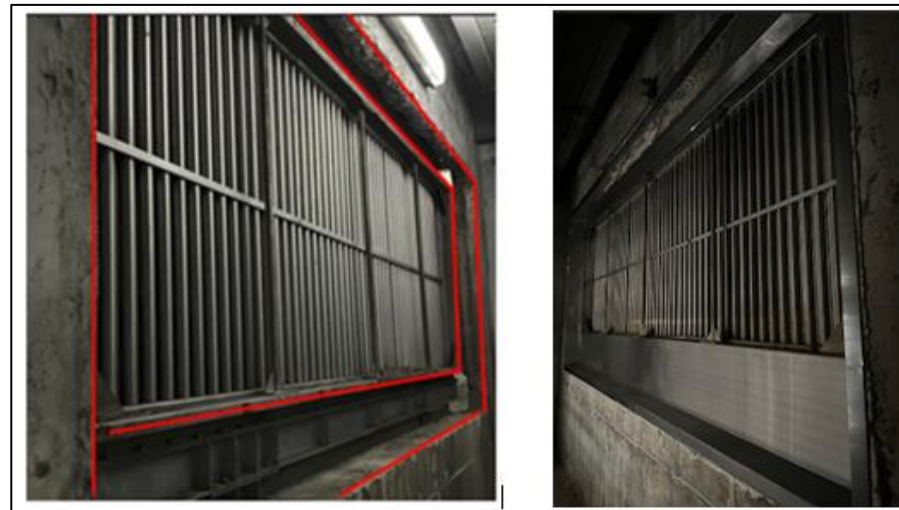
CASE3. Insulation of the leakage at Heat exchanger (Problems of leakage air)
