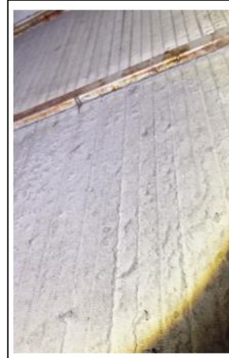
CASE2. Improved air flow with cleaning of the plugged filter for the supply air V2906
