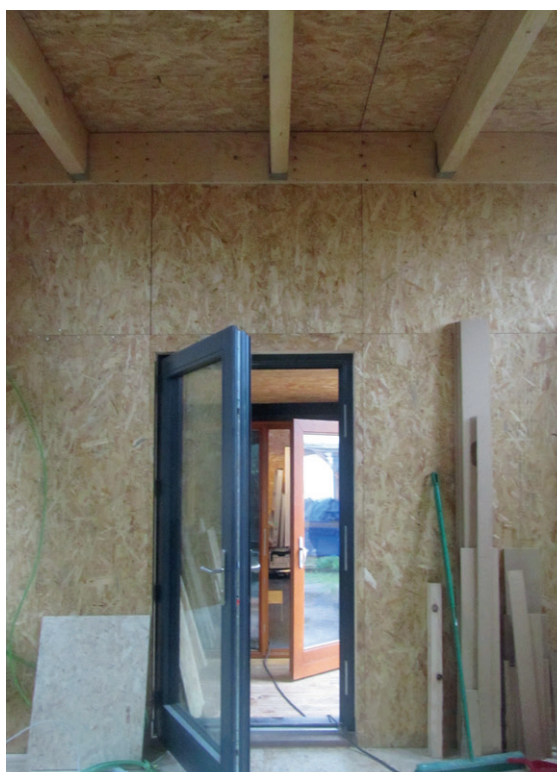
Mock-up of low energy house: EFB Vocational Training College, Brussels
