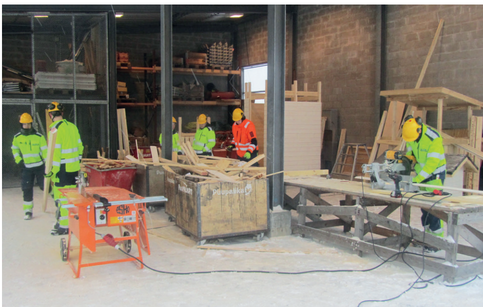
Carpentry workshop: Vantaa Vocational College, Varia/Finland
