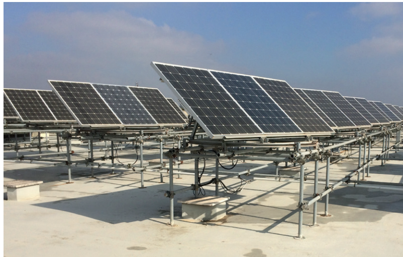
Solar panels used for training and supplying electricity to CEFME CTP training centre for Rome province
