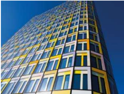
Facade and fenestration manufacture
