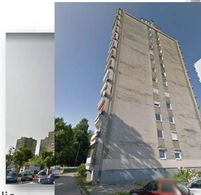
Vir: Google Street View
